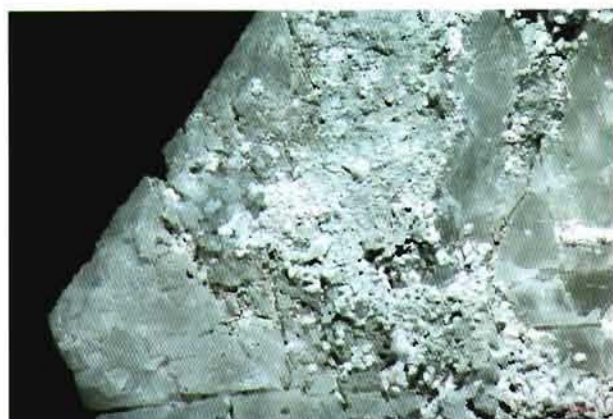
Figure 4. The bottom left hand side of Fig. 3, showing the deep corrosion of the baryte.
